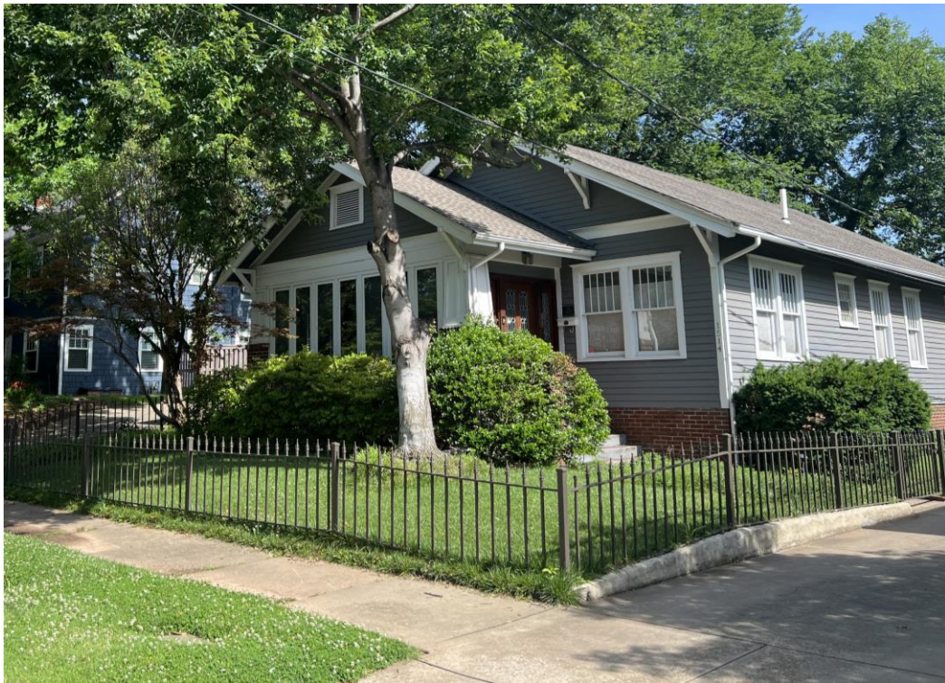
1514 East 17 th Place – Present (view southeast)
