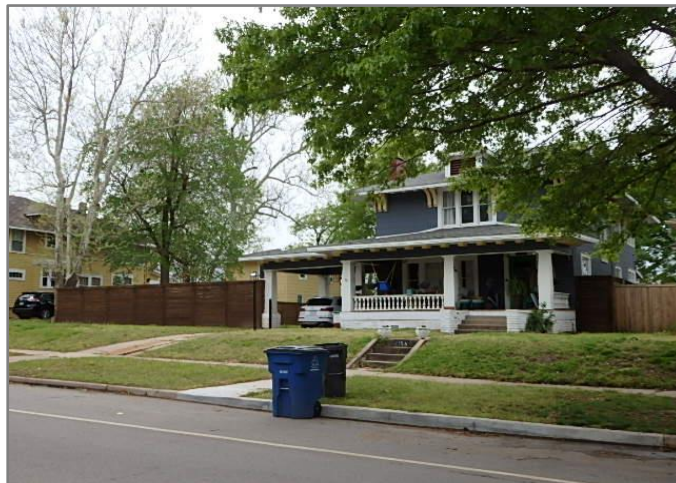
1156 North Denver Avenue – View Southwest
