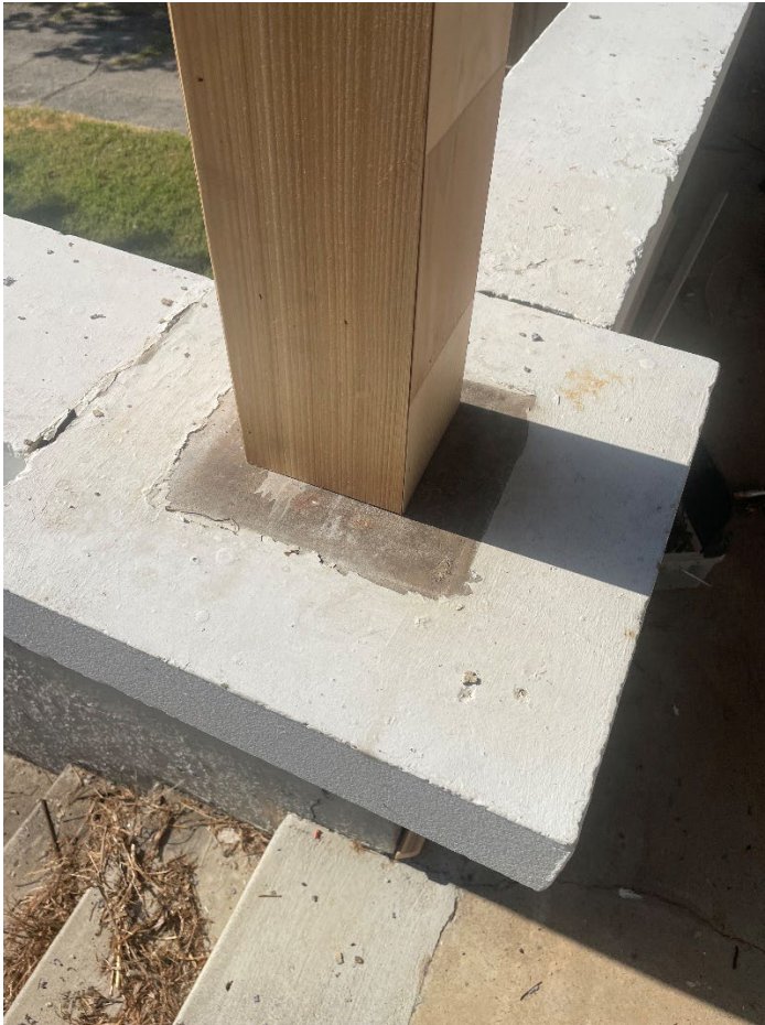
Newly installed porch columns (picture provided by the applicant)
