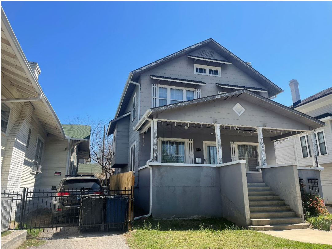
(Picture provided by applicant)
