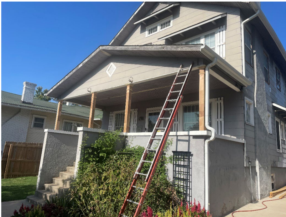
Newly installed 4-inch by 4-inch porch columns (picture provided by the applicant)
