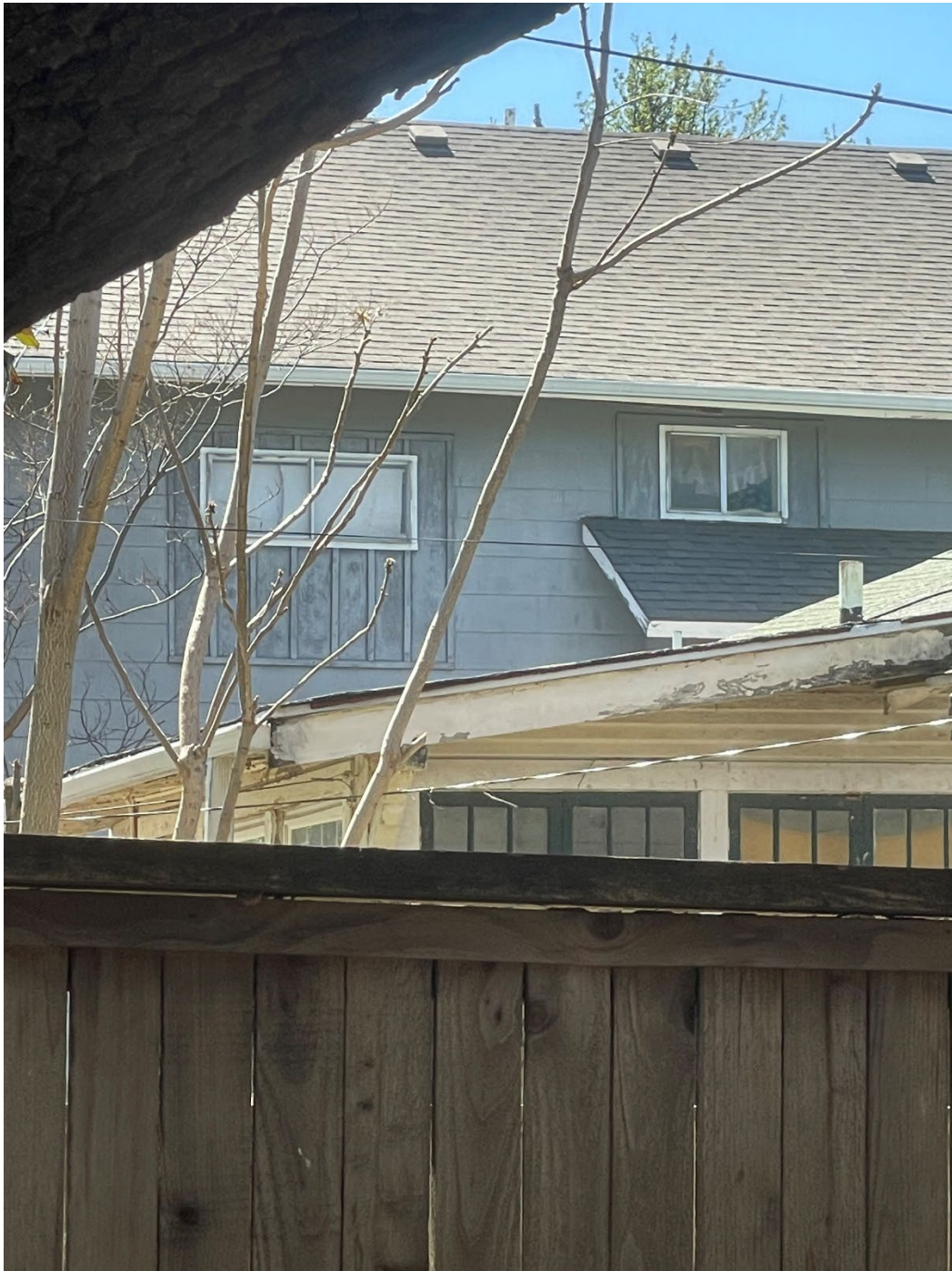
Proposed window to be replaced on the North side of the residence (picture provided by the applicant)
