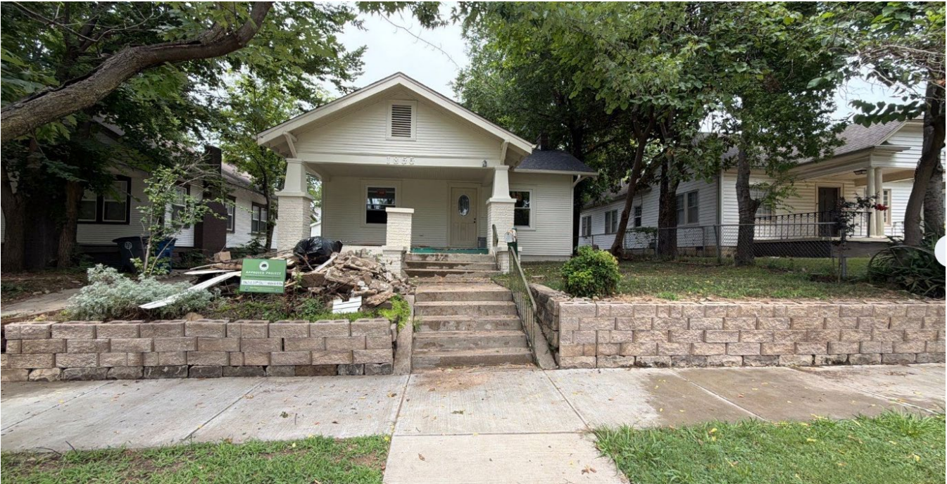
Newly constructed wall, image provided by applicant
