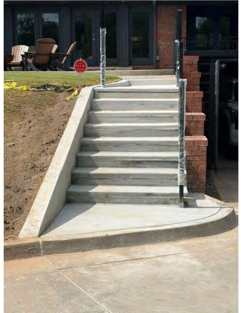
New concrete steps and bulkhead
