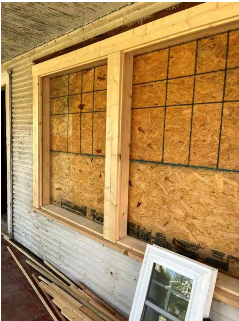
Mockup of window trim
