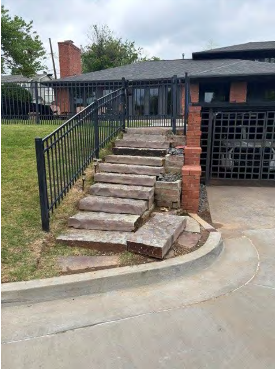
Previous stone steps and rail
