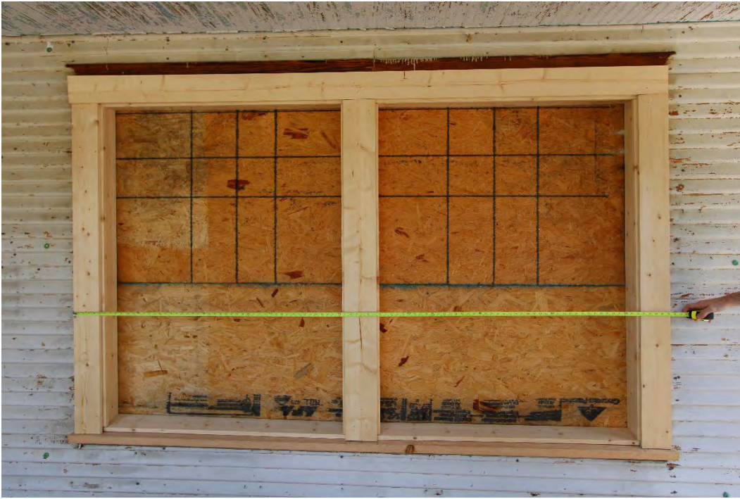
Mockup of window trim
