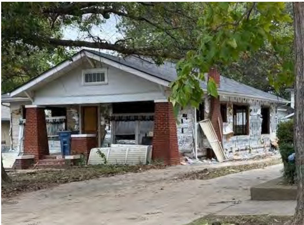
Work in progress, October 2026
