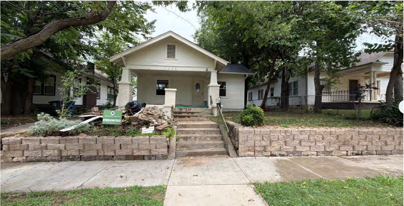
Newly constructed wall, image provided by applicant
