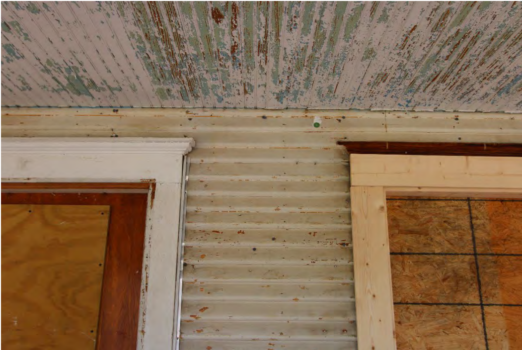
Crown moulding on window (previous) and door (current)
