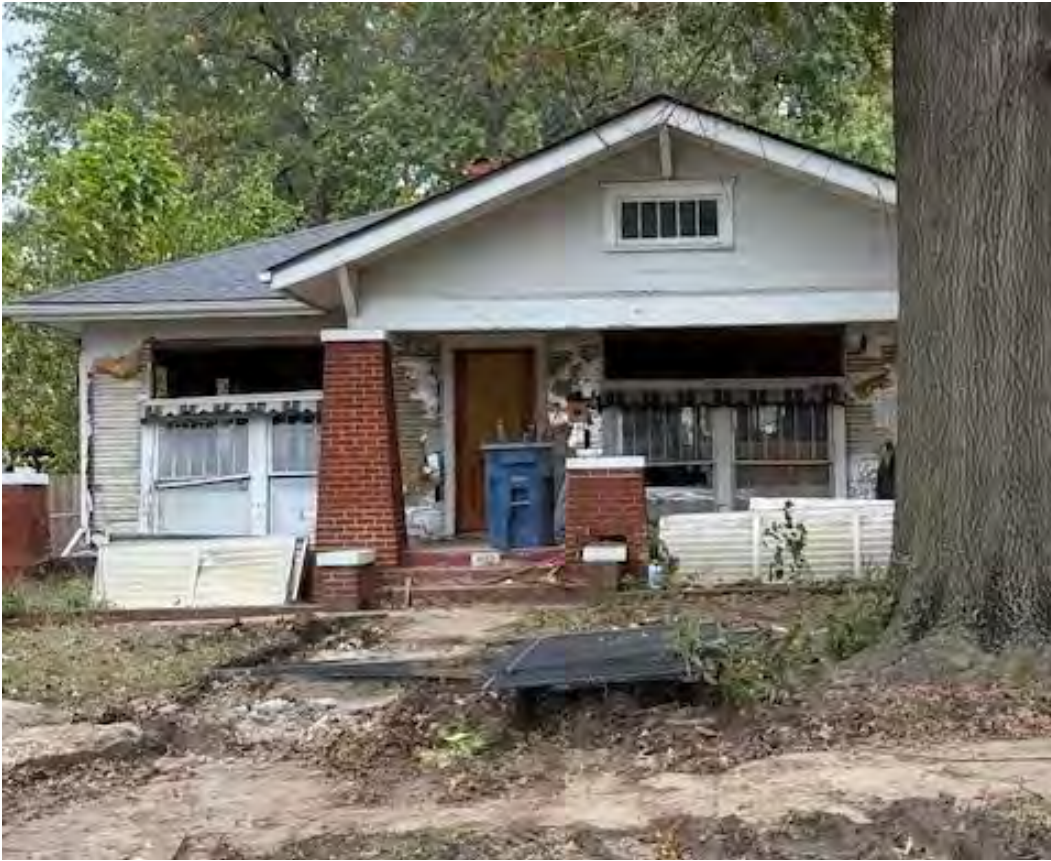
Work in progress, October 2026
