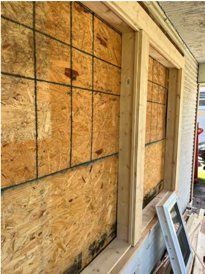
Mockup of window trim
