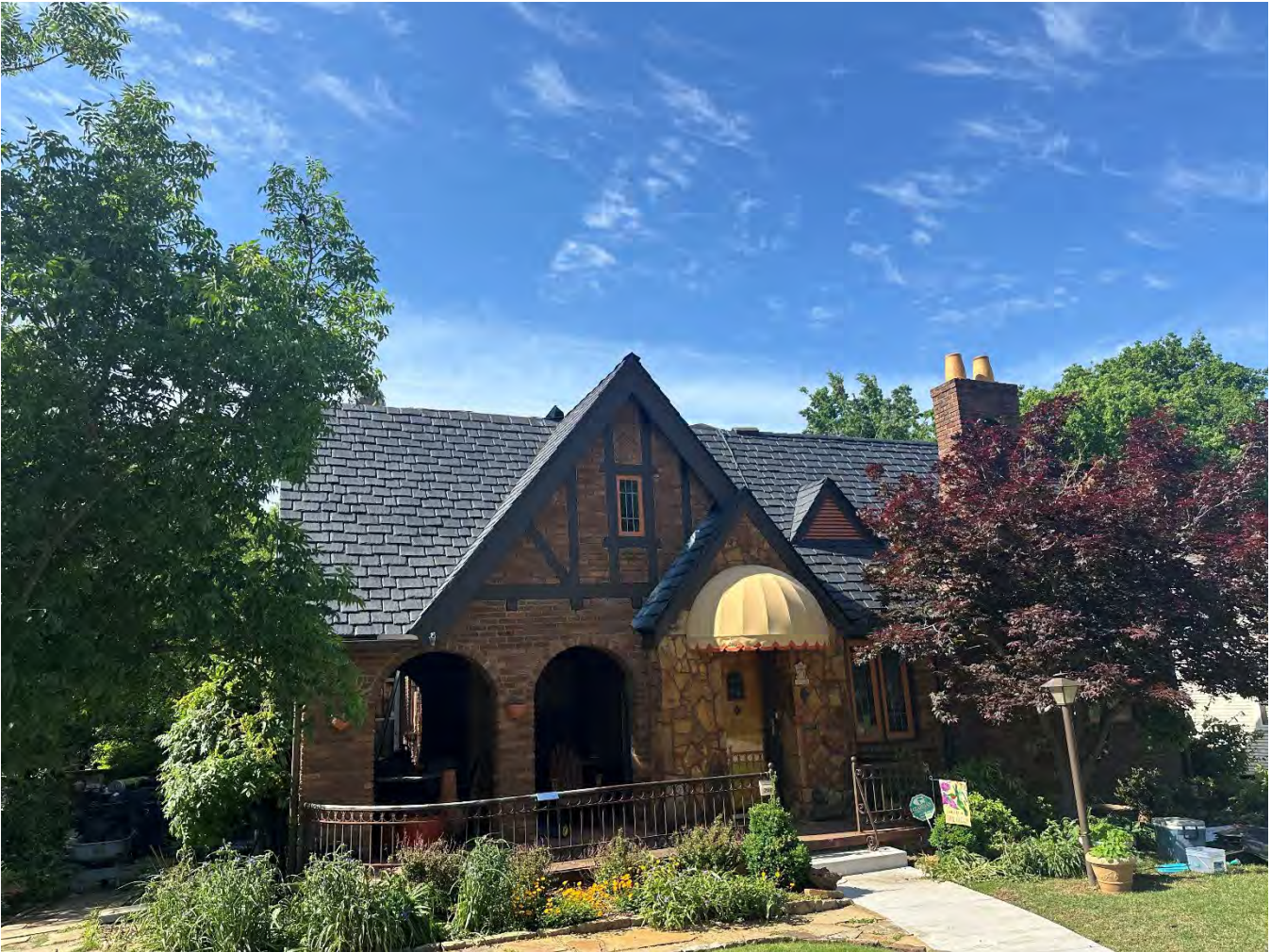
2224 E. 20 th St – Recent installation nearby with Da Vinci composite slate roof
