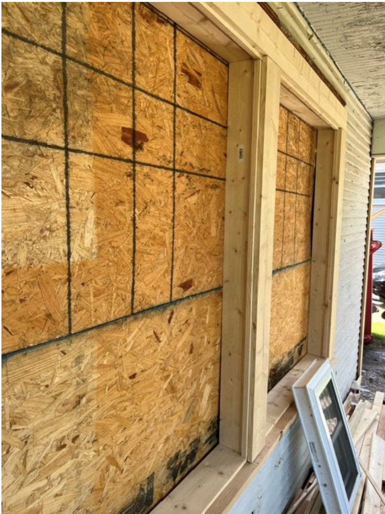
Mockup of window trim
