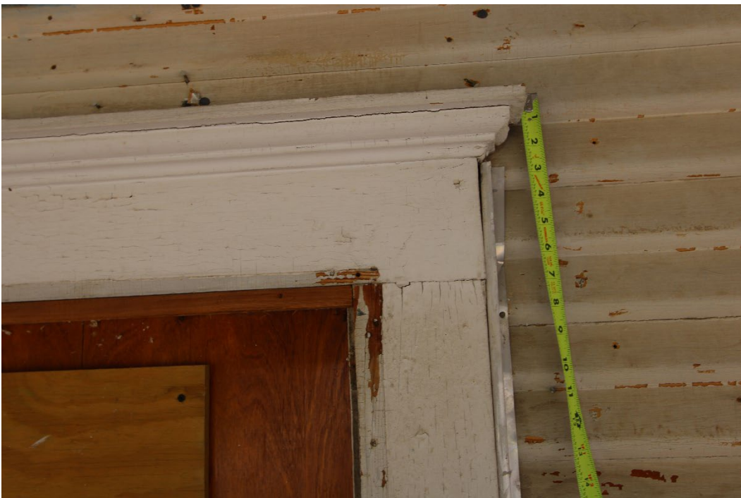
Crown moulding on door
