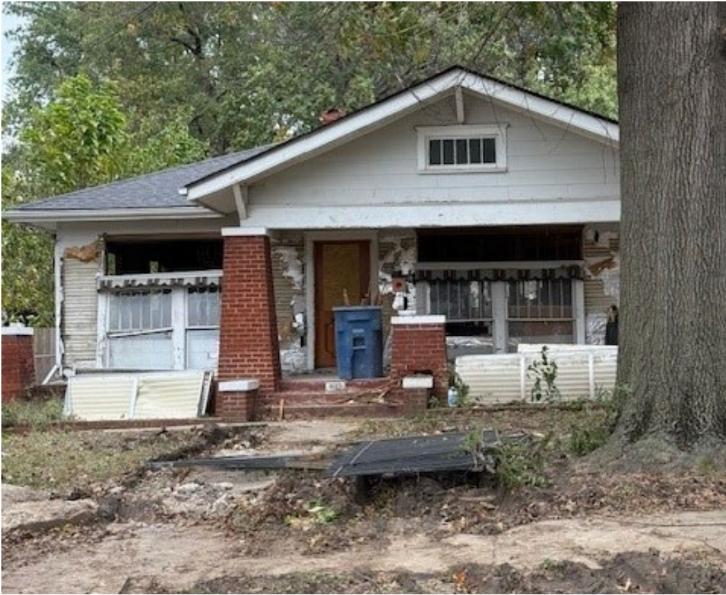
Work in progress, October 2026
