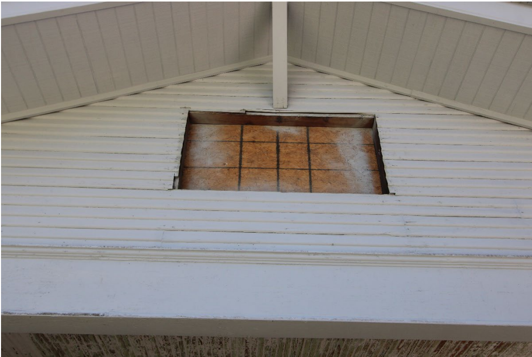
Porch gable window opening
