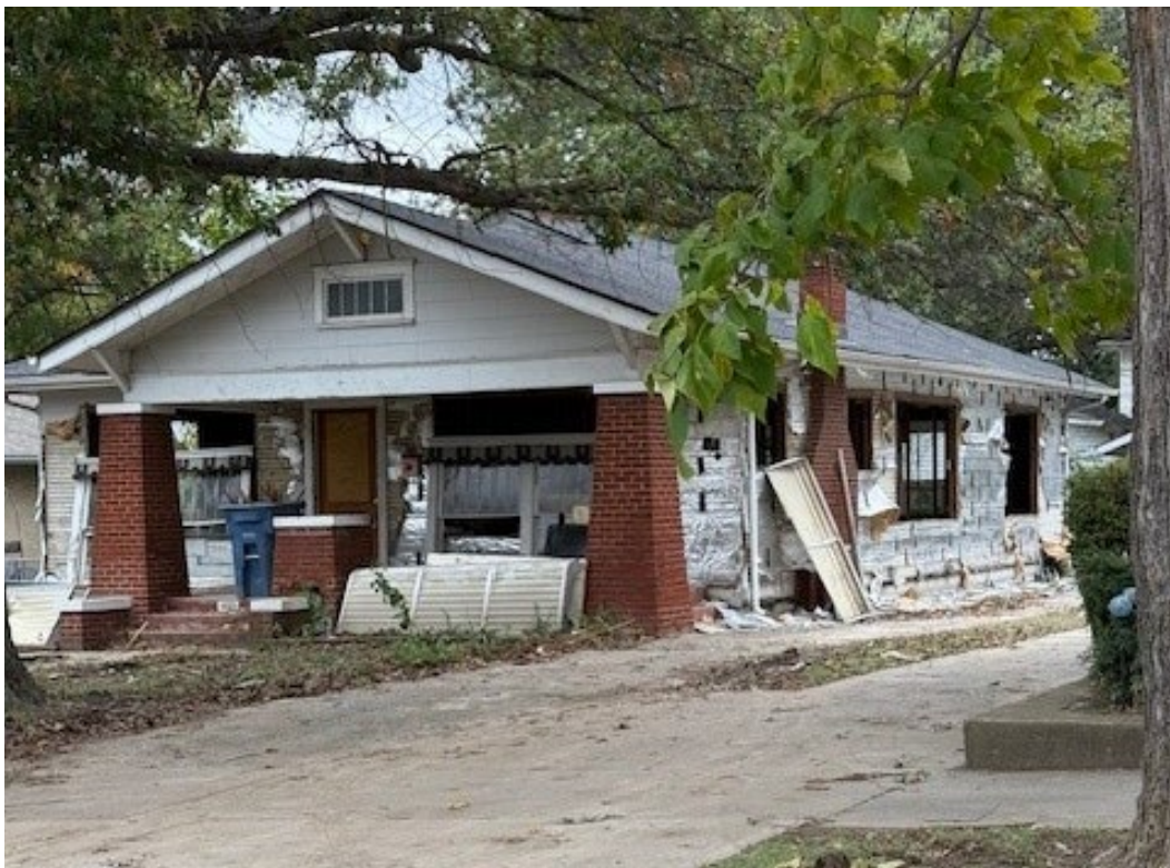
Work in progress, October 2026
