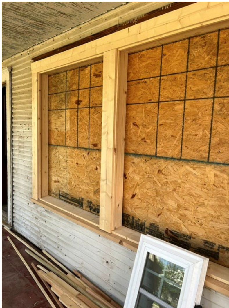
Mockup of window trim
