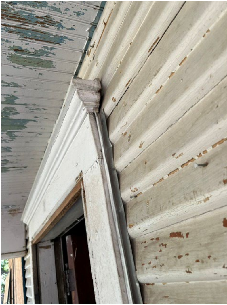
Crown moulding on door
