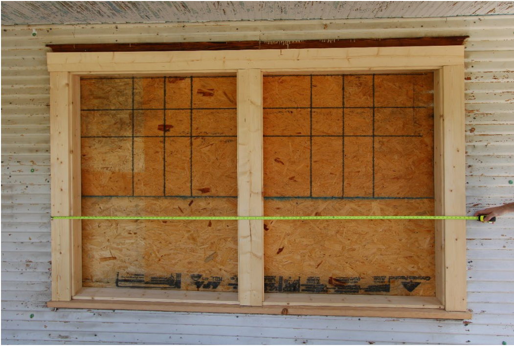
Mockup of window trim
