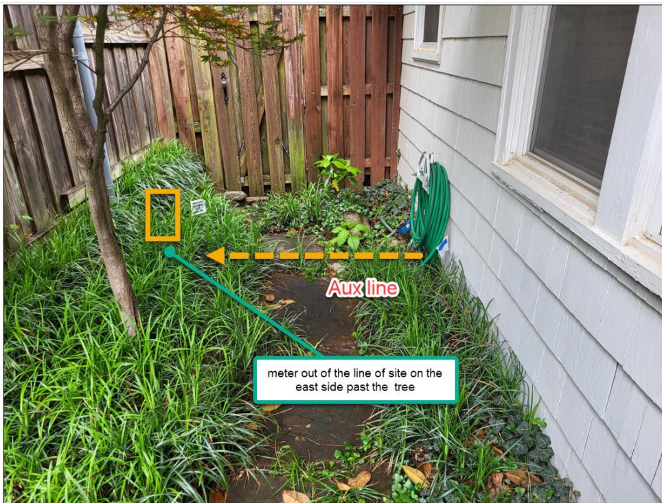
Location of new meter
