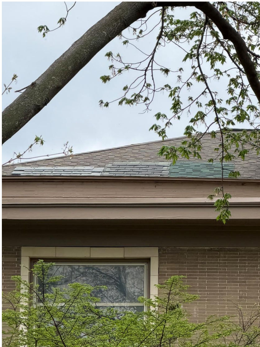
Roof with DaVinci samples
