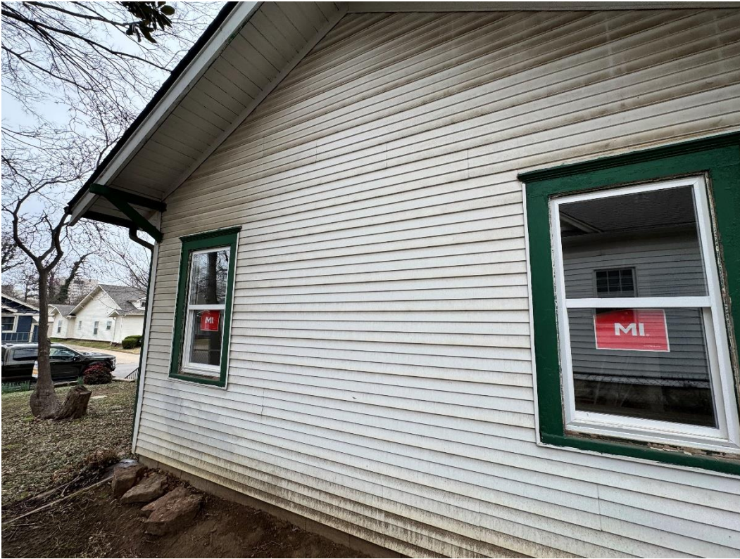
East side of residence
