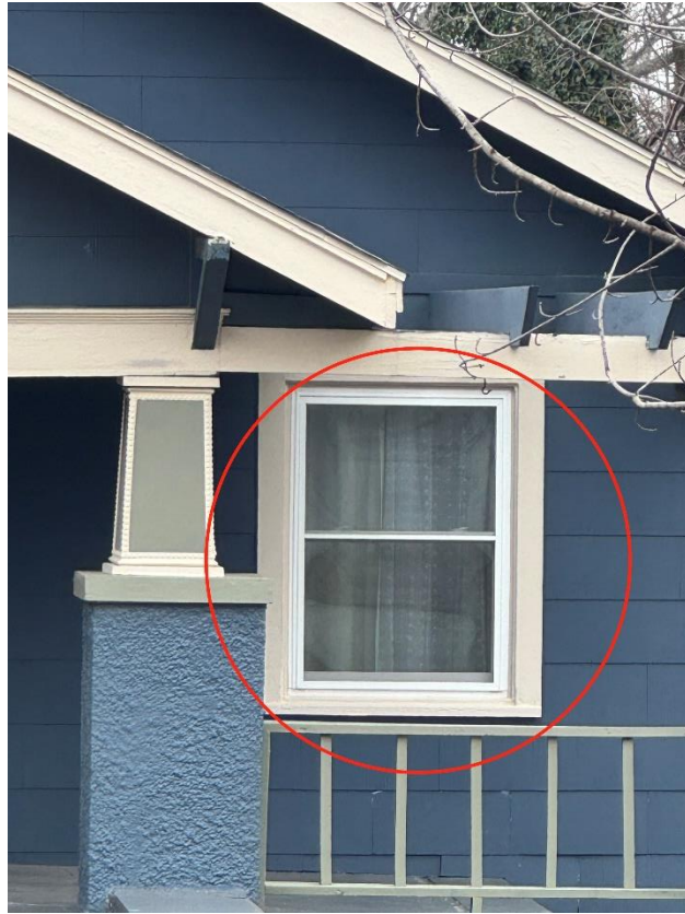
Neighborhood example of window
