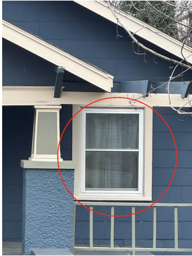
Neighborhood example of window
