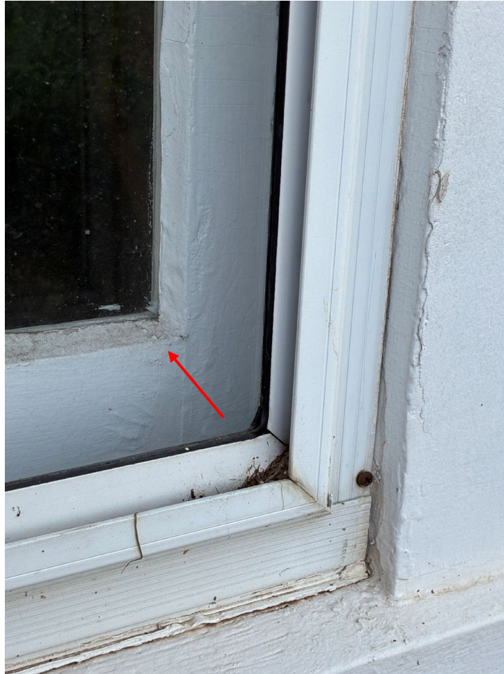
Example of beveled edge on window profile
