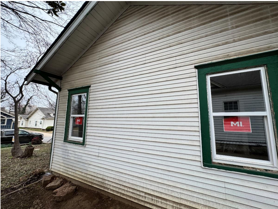
East side of residence
