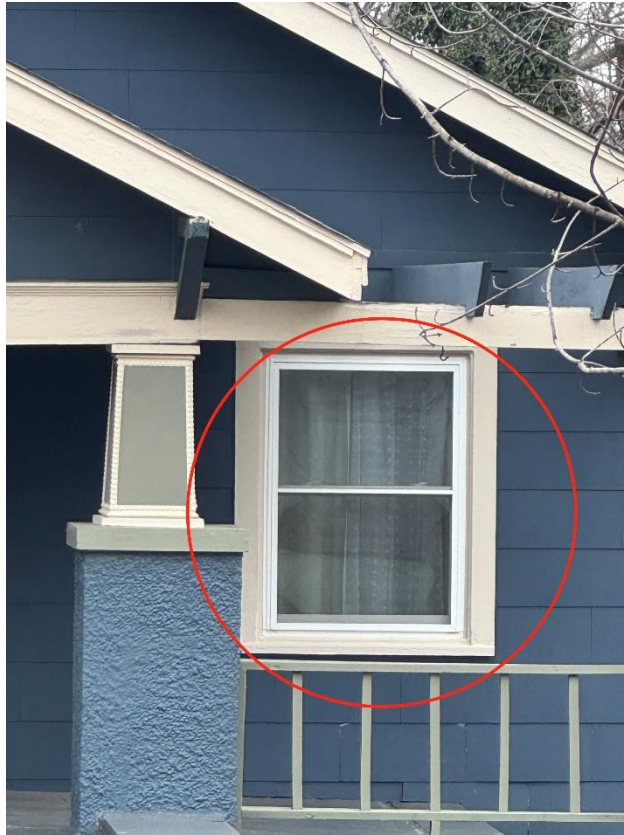
Neighborhood example of window
