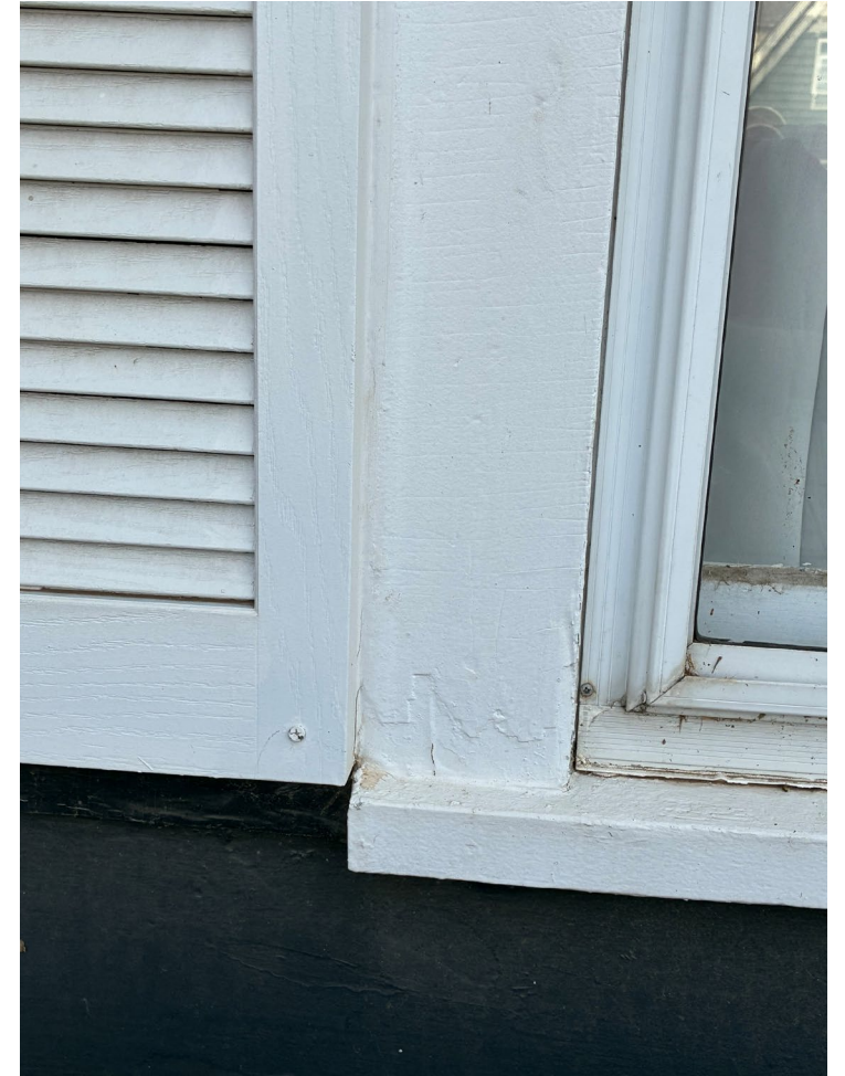
Example of window sill
