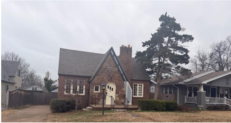
front side of the house- 1
