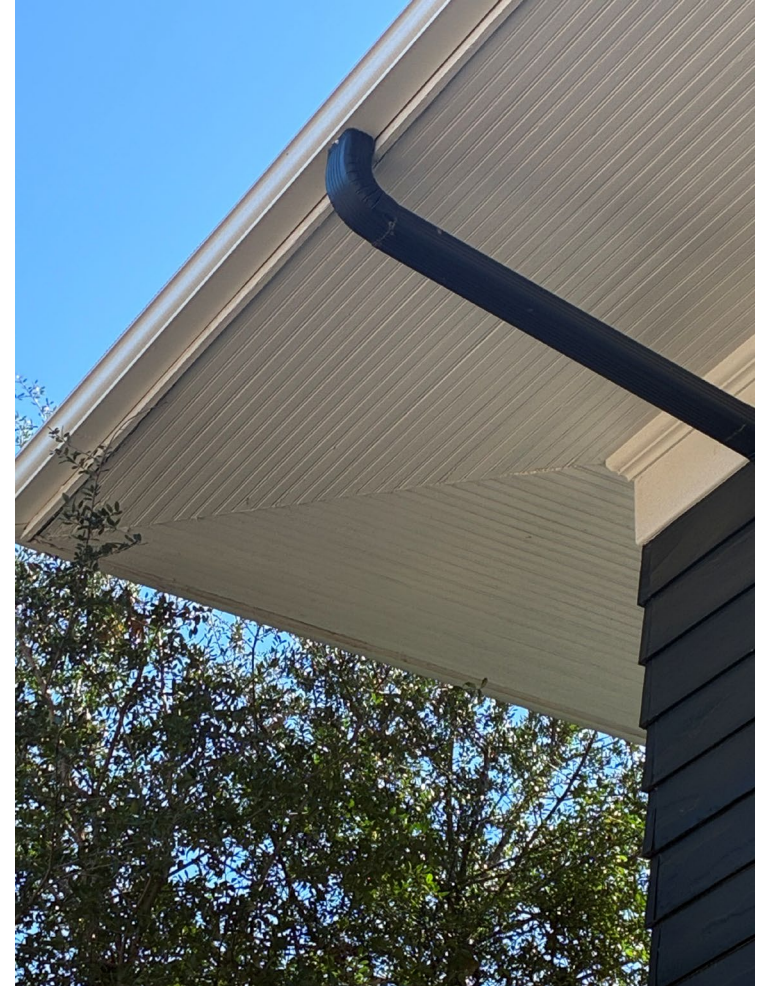
Soffit material: match existing
