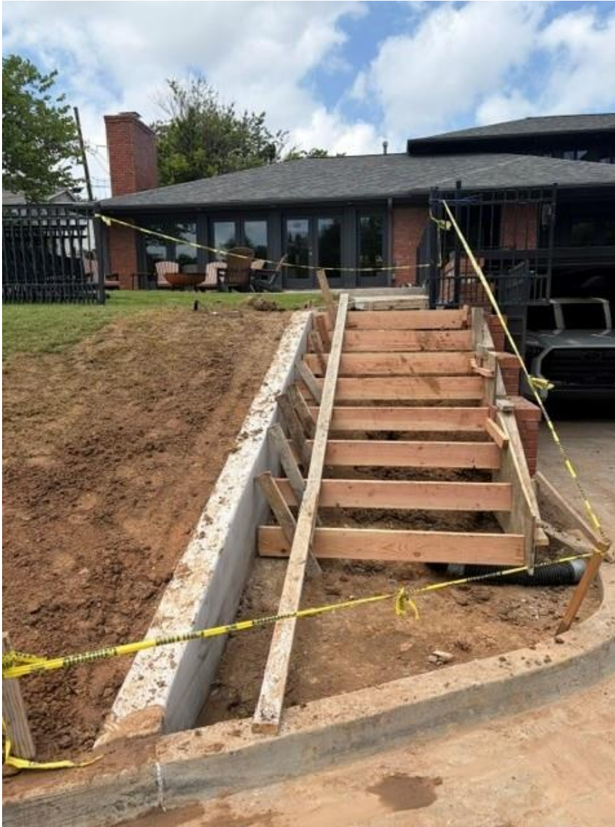
Steps in progress
