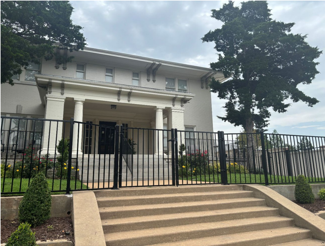
View south from street
