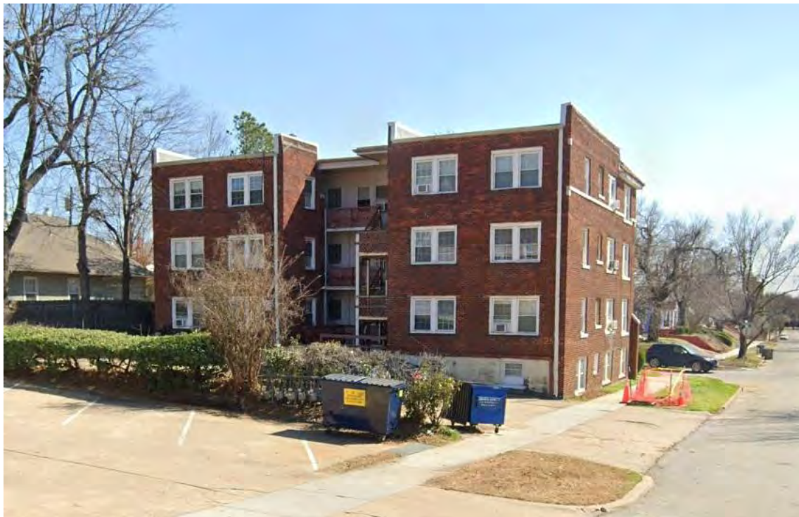
Rear (north) of building, view southeast from Quaker Avenue
