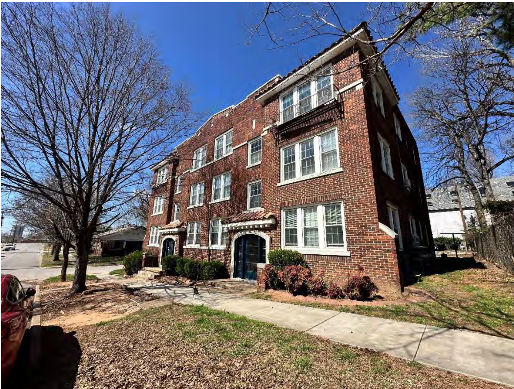
Front (south) side of building, view northwest from 17th Street
