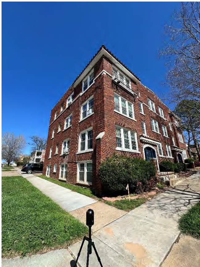
Front (south) and west side of building, view northeast from 17th & Quaker intersection
