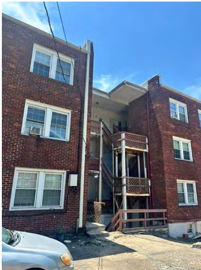
Staircase on north side of building
