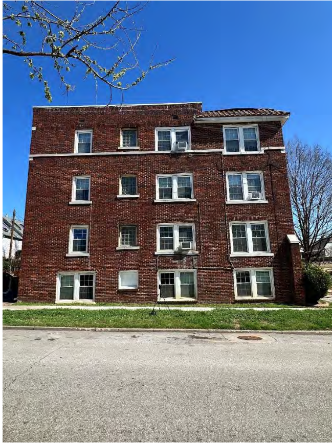
West side of building, view east from Quaker Avenue
