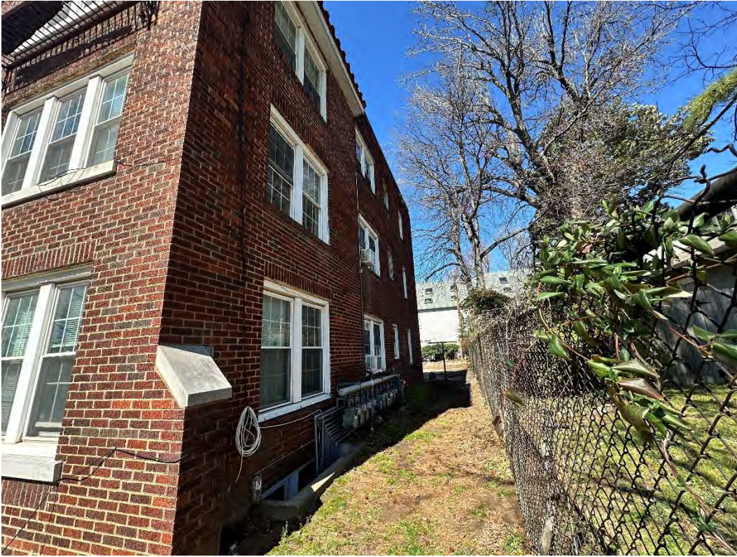
East side of building, view north/northwest
