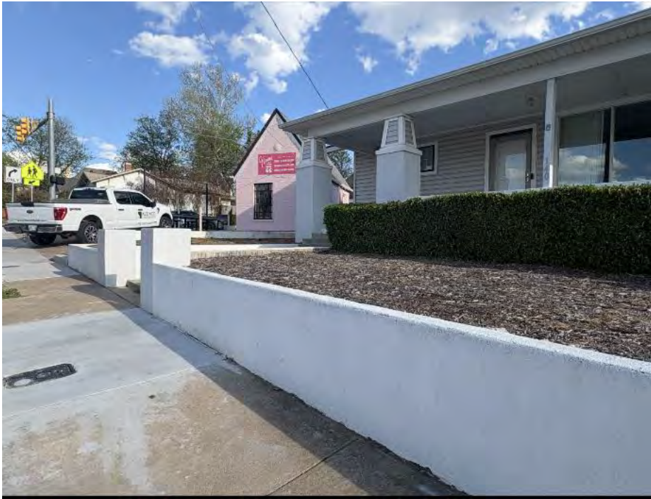
Example from 140 East 18th Street
