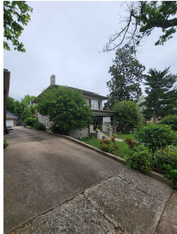
LOOKING NORTHEAST FROM SIDEWALK AT WEST NEIGHBOR'S DRIVEWAY
