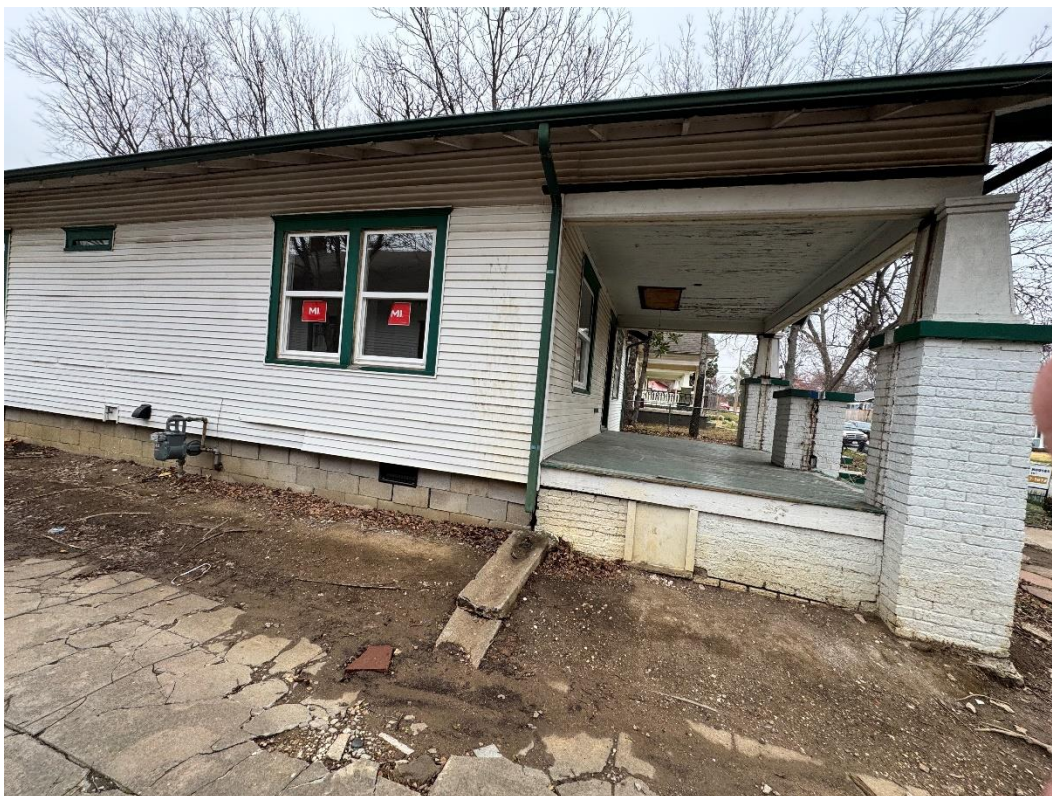
West side of residence
