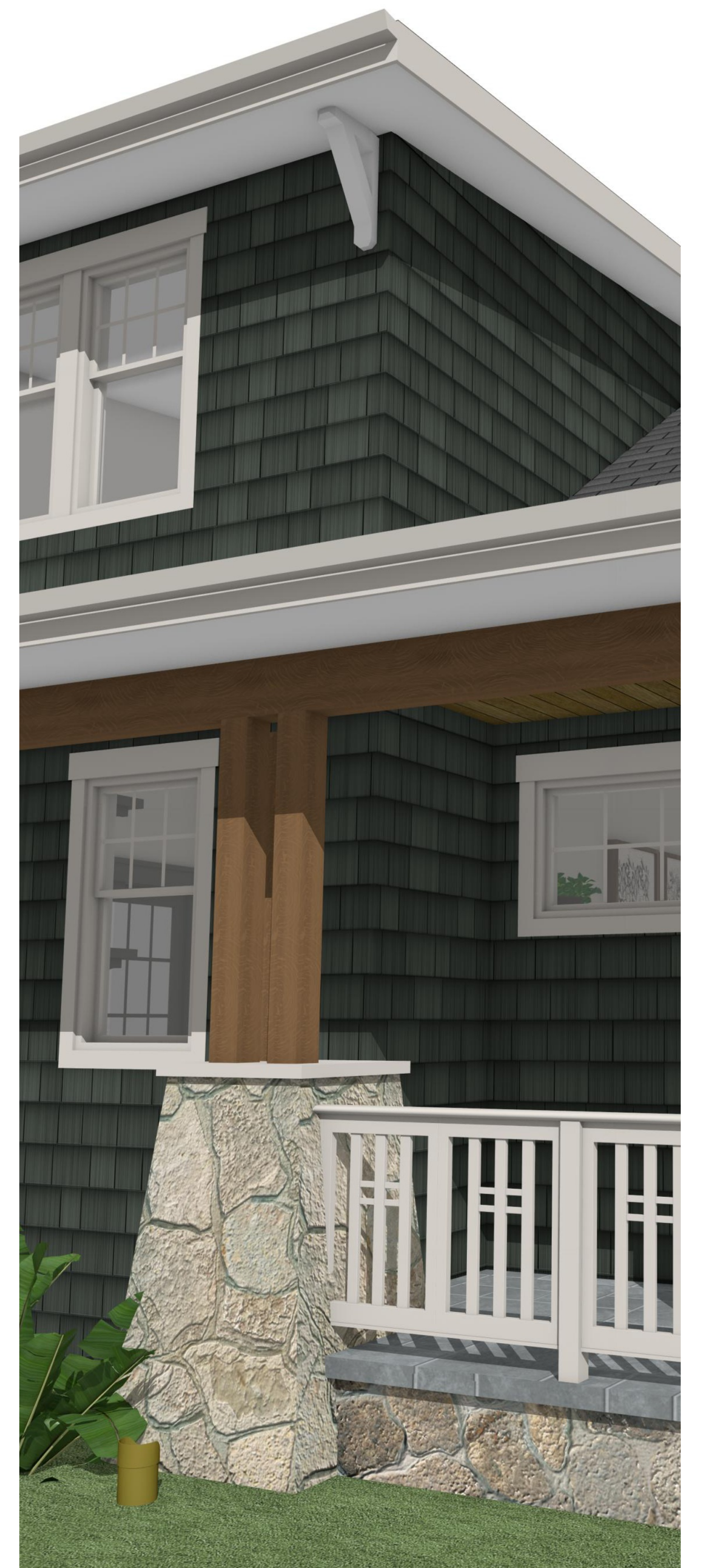
KNEE BRACE EAVE DETAILS AND COLUMN
