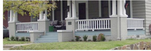
Traditional design with railing lower than piers
