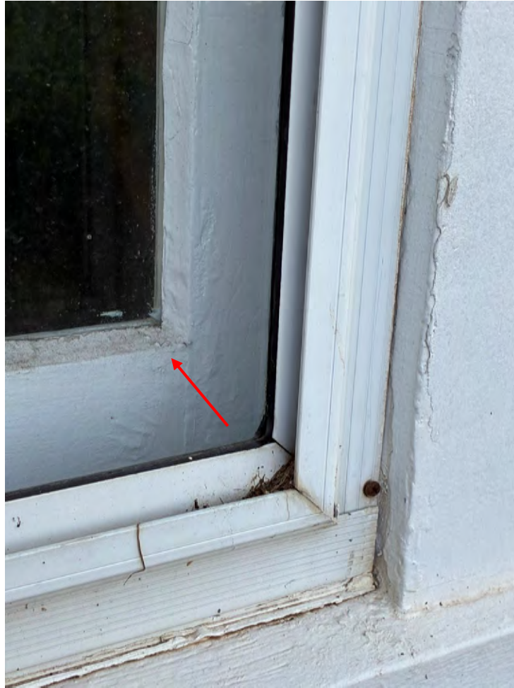
Example of beveled edge on window profile
