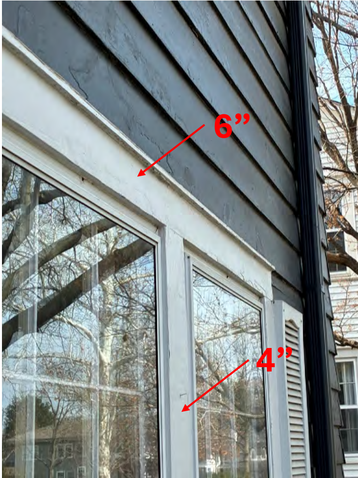
Example of 1x4 flat trim on window
