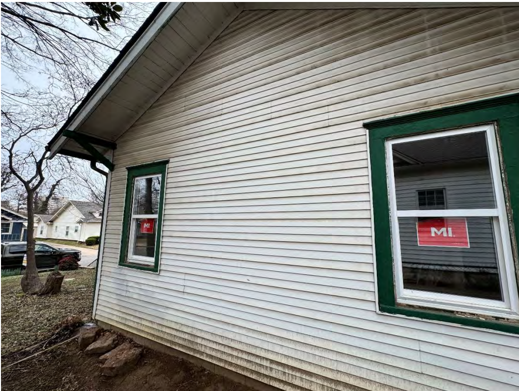
East side of residence
