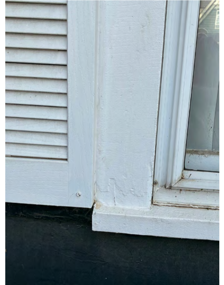
Example of window sill
