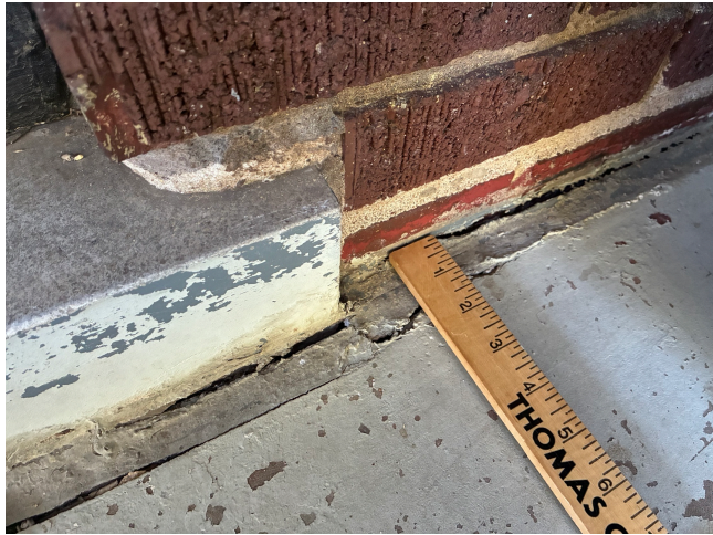
East Patio - Separation Damage
