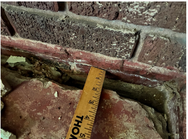
North Patio - Separation Damage
