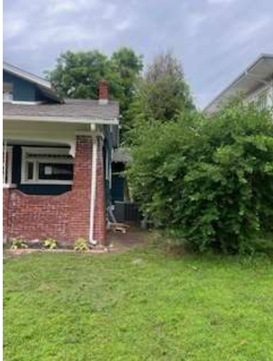
Side of home (north)
