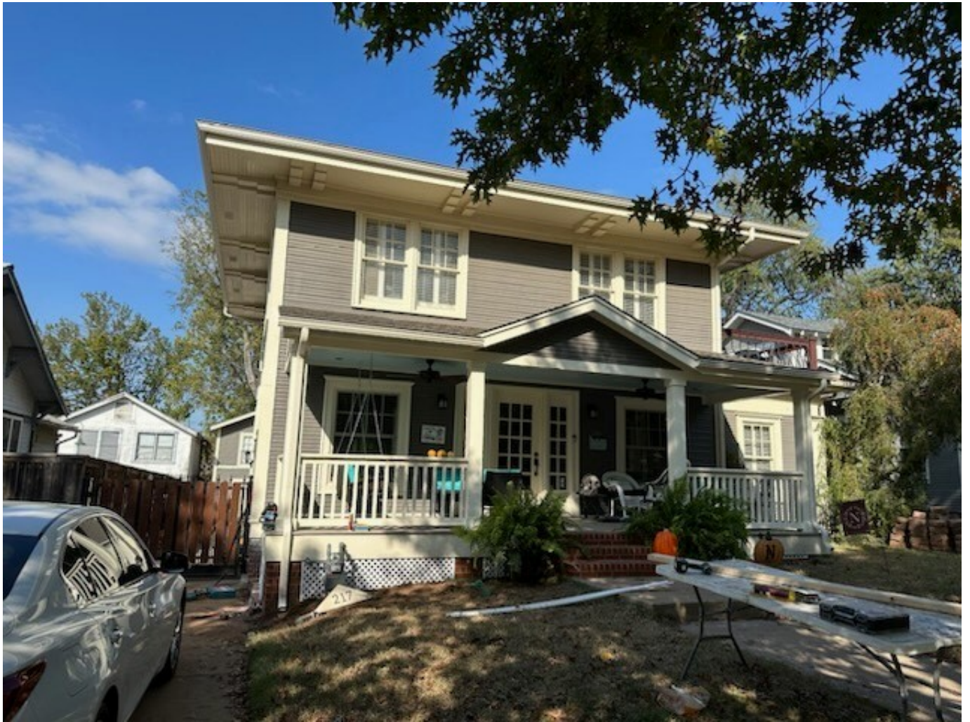
View from the South; Railing Height is 36"
