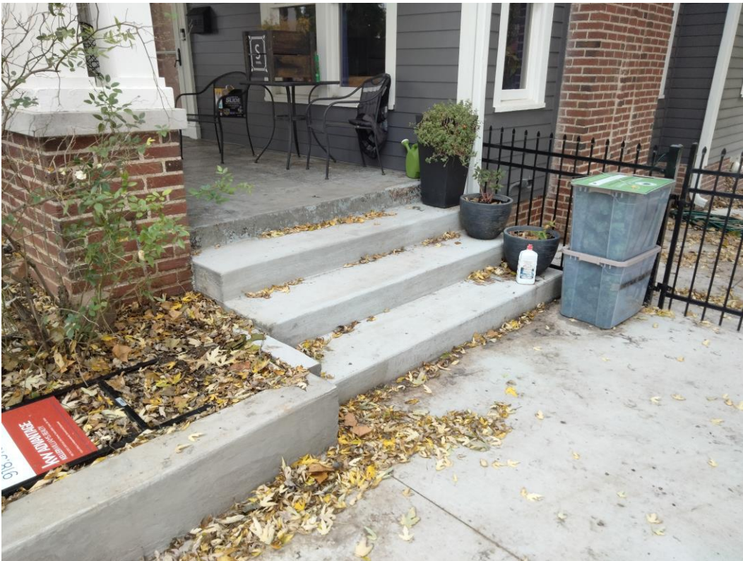
Steps after replacement
