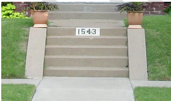
G.2.1 Bulkheads are the sloped strips of paving flanking the steps above. Note the width of the paving and how the angle is flush with the sidewalk, not raised above it.
