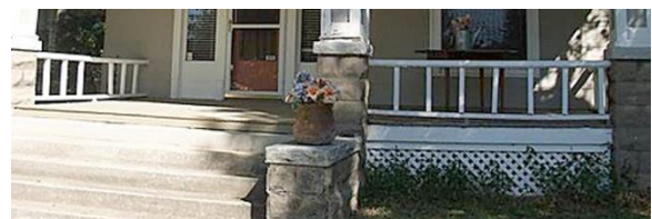
Inappropriate design – balusters too far apart.
