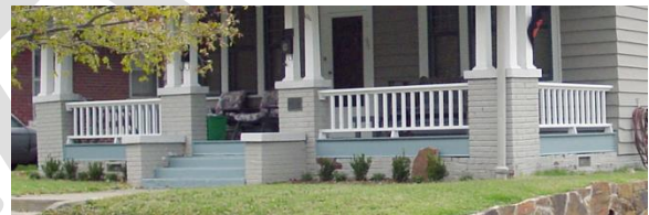
Traditional design with railing lower than piers.
