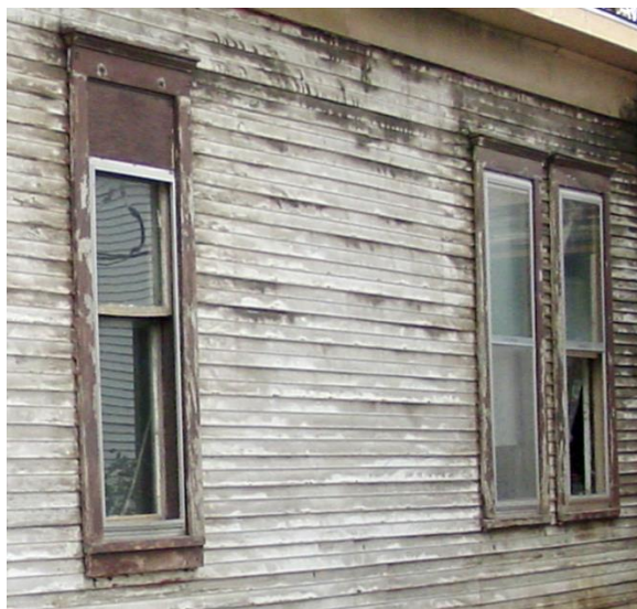
A.4.5 Inappropriate resizing, left window opening
