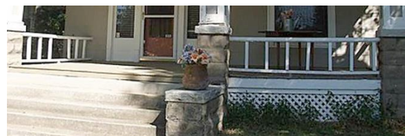
Inappropriate design – balusters too far apart.
