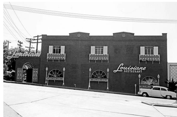
A.1.1 Before (left) and after (right) photographs of historic architectural elements lost during rehabilitation of a Plains Commercial building. Without the original window pattern, storefronts, transom windows, and pad stone insets at the upper corners of the second-floor windows, the building loses its historic character.
