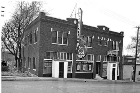
A.1.1 Before (left) and after (right) photographs of historic architectural elements lost during rehabilitation of a Plains Commercial building. Without the original window pattern, storefronts, transom windows, and pad stone insets at the upper corners of the second-floor windows, the building loses its historic character.
