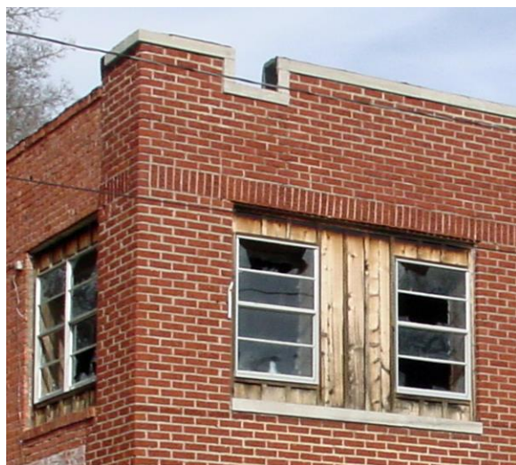
A.4.5 Inappropriate resizing of window openings
