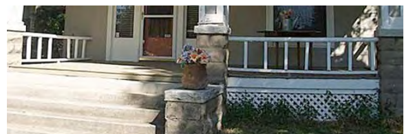
Inappropriate design – balusters too far apart.
