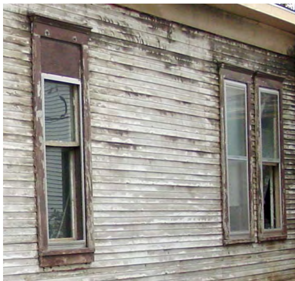
A.4.5 Inappropriate resizing, left window opening
