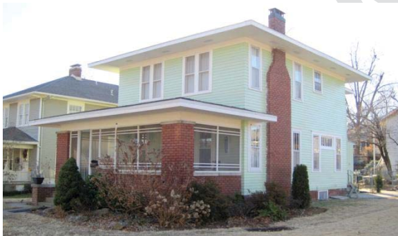
B.5.2 Example of enclosing a front porch with screens that maintains the character of the Prairie style house and can be removed in the future without damaging the historic brick columns.
