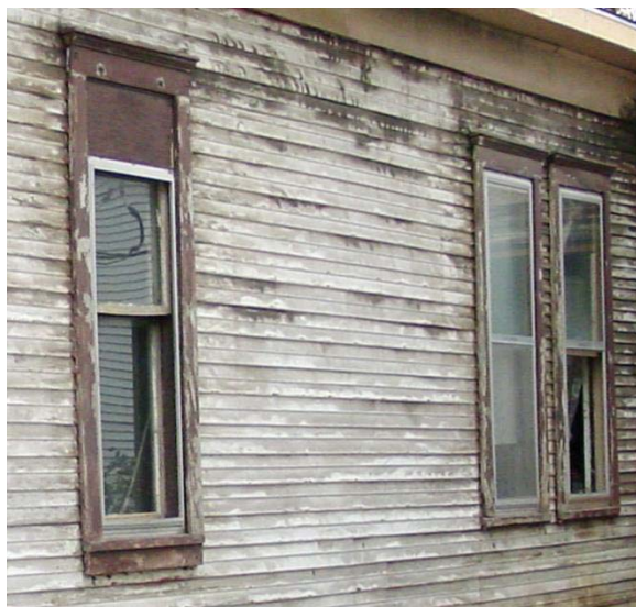
A.4.5 Inappropriate resizing, left window opening
