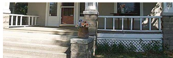
Inappropriate design – balusters too far apart.
