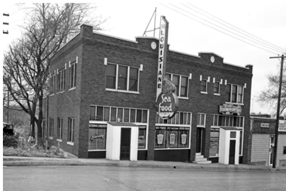
A.1.1 Before (left) and after (right) photos of historic architectural elements lost during rehabilitation of a Plains Commercial building. Without the original window pattern, storefronts, transom windows, and pad stone insets at the upper corners of the second floor windows, the building loses its historic character.
