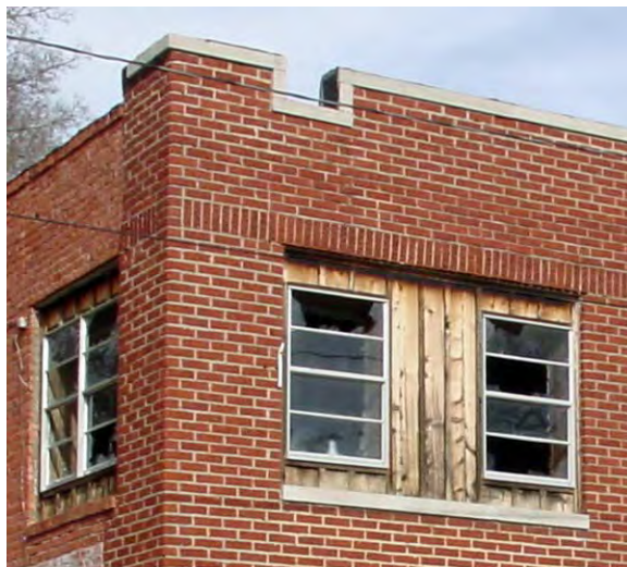
A.4.5 Inappropriate resizing of window openings
