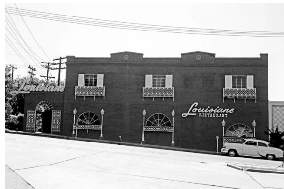
A.1.1 Before (left) and after (right) photos of historic architectural elements lost during rehabilitation of a Plains Commercial building. Without the original window pattern, storefronts, transom windows, and pad stone insets at the upper corners of the second floor windows, the building loses its historic character.
