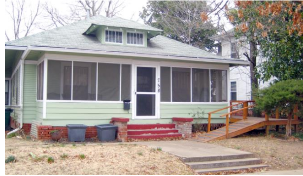
B.5.3 Example of a ramp for accessibility that enters the front porch from the side. The ramp can be easily removed in the future without needing to repair the historic materials on the front elevation.
