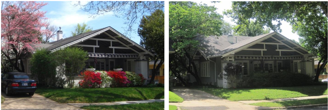
B.4.2 On the left is a house before an addition to the side elevation. On the right is the same house with an addition to the side elevation matching the proportions and rhythm of the existing roof line.
