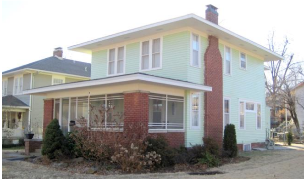
B.5.2 Example of enclosing a front porch with screens that maintain the character of the Prairie-Style house and can be removed in the future without damaging the historic brick columns
