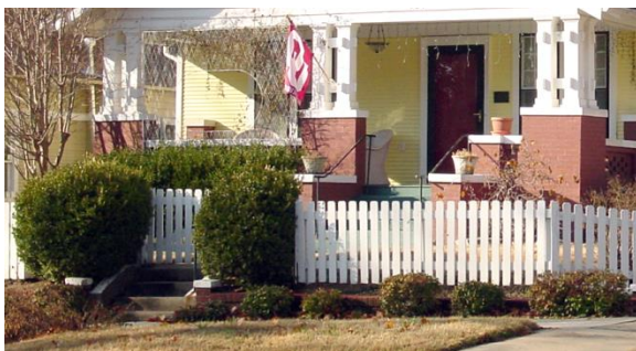
G.1.4 Low wooden picket (and, in some instances, wrought-iron) fences are most appropriate.
