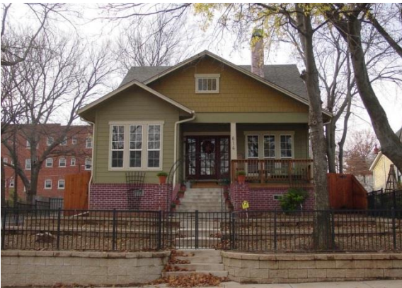
C.1.1 / C.1.2 While not a duplicate of existing houses, this house draws upon common characteristics of the district—raised crawl space, front porch, multiple front gables, siding patterns, and groups of windows.
