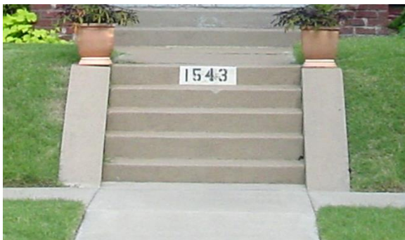
G.2.1 Bulkheads are the sloped strips of paving flanking the steps above. Note the width of the paving and that it is flush with the sidewalk and not raised above it.
