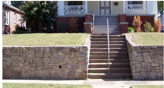
G.1.5 Historically, retaining walls were constructed of native stone or brick.
