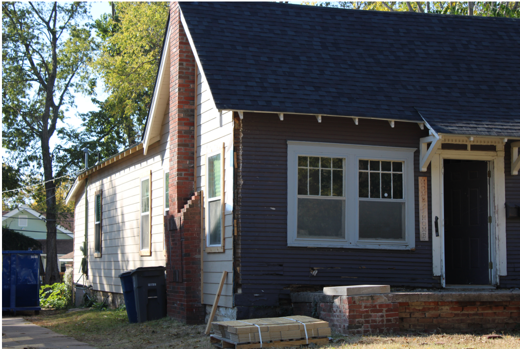
Installation of 8" Lap and rough cedar trim
