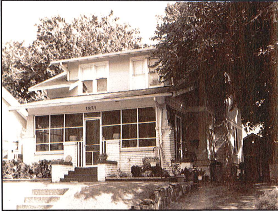
1851 East 17 th Street – Survey Photograph – July 11, 2007
