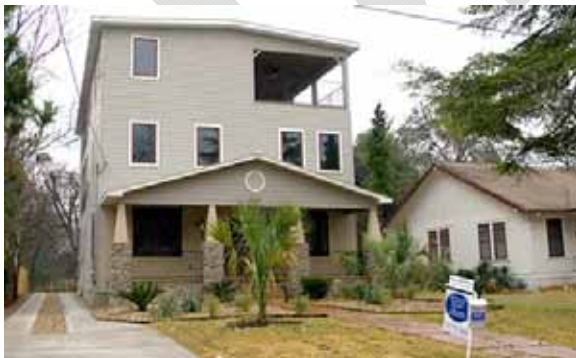
B.1.4 Example of an addition that doesn't respect the height of structures on same street.
