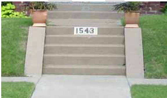
G.2.1 Bulkheads are the sloped strips of paving flanking the steps above. Note the width of the paving and how the angle is flush with the sidewalk, not raised above it.
