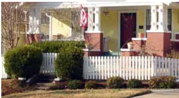
G.1.4 Low wooden picket (and, in some instances, wrought iron) fences are most appropriate.
