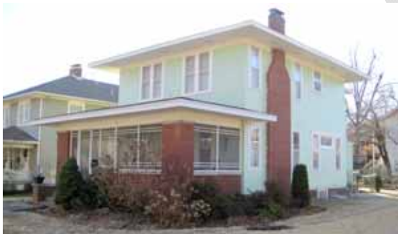
B.5.2 Example of enclosing a front porch with screens that maintains the character of the Prairie style house and can be removed in the future without damaging the historic brick columns.
