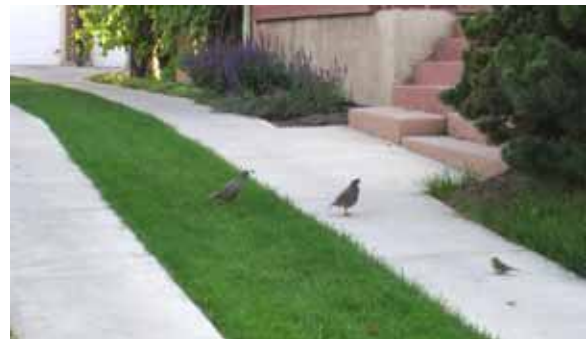
G.2.2 Historically, driveways in Tulsa were plain concrete slabs. A great alternative is the ribbon driveway (above), which uses less concrete, creates less runoff, and is historically appropriate.
